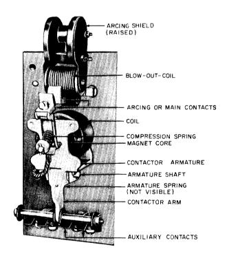
Fig. 1—Typical Contactor
