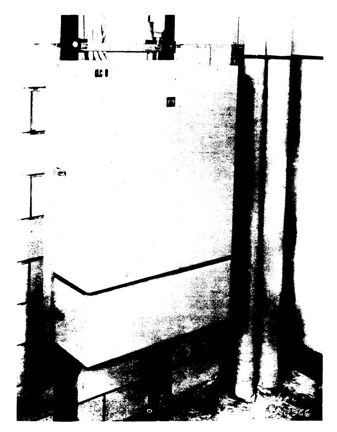
Fig. 1 — Gfeller Line Concentrator 49-9-2 Mounted Central Office Unit
