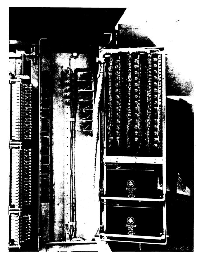
Fig. 7 – Gfeller Line Concentrator 49-9-2 Remote Unit (Interior View, Relay Rack Gate Open)
