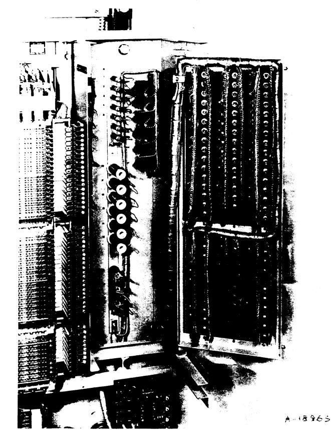
Fig. 5 — Gfeller Line Concentrator 49-9-2 Central Office Unit (Interior View, Relay Rack Gate Open)
