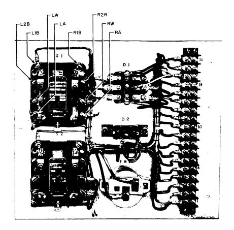
Fig. 18 – Control Panel — S1 Relay Terminal Designations — 659A, 659B, and 659C Wiring Shown
