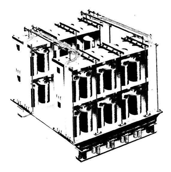
Fig. 9-Polyester Glass Battery Stand With Cells Mounted on Shock Isolation Platform in Hardened Site
