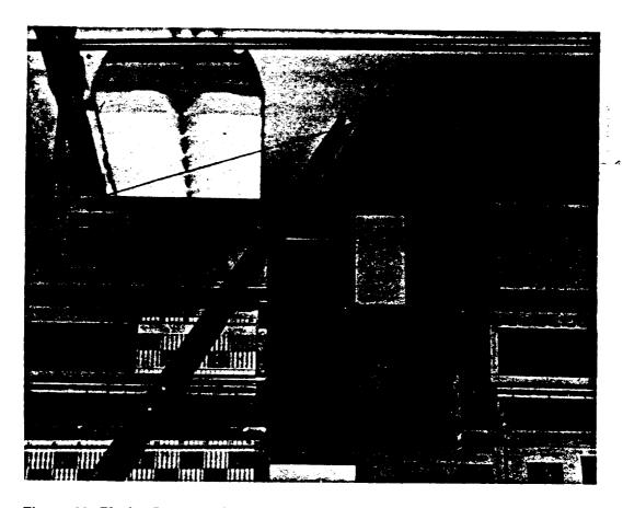
Figure 32. Placing Jumper Wire in Trough Using Jumper Running Tool
