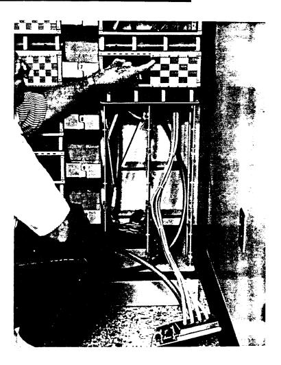
Figure 21. Mounting of 112-Type Block Assembly on Mini COSMIC Frame (Front View)
