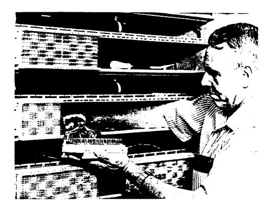
Figure 17. Connecting Block Being Placed in Frame
