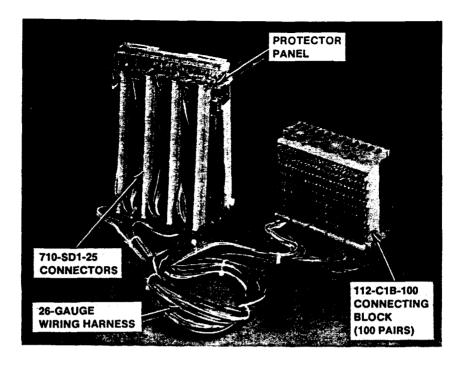
Figure 10. 307D1-100 Connector — Back View
