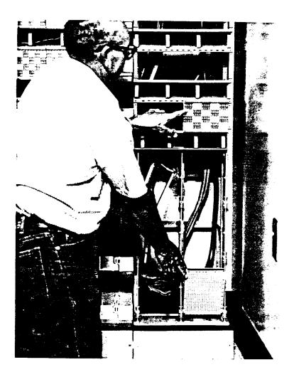
Figure 22. Routing UL Connector Stub Cable on Mini COSMIC Frame (Front View)
