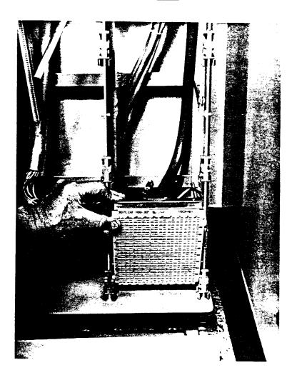
Figure 24. Latching UL Connector Panel on Mini COSMIC Frame
