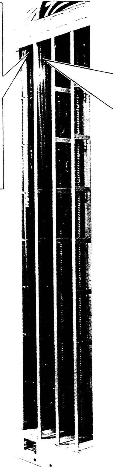
Figure 7—Dressing and Securing Stub Cable in MPF Verticals—Rear View
