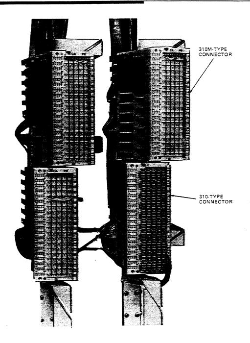
Figure 1. Angle Mounted 310M-Type (Top) and 310-Type Connector (Bottom) [Extends 7 Inches (17.78 cm) from Face of Vertical Frame Mounting Bar.]
