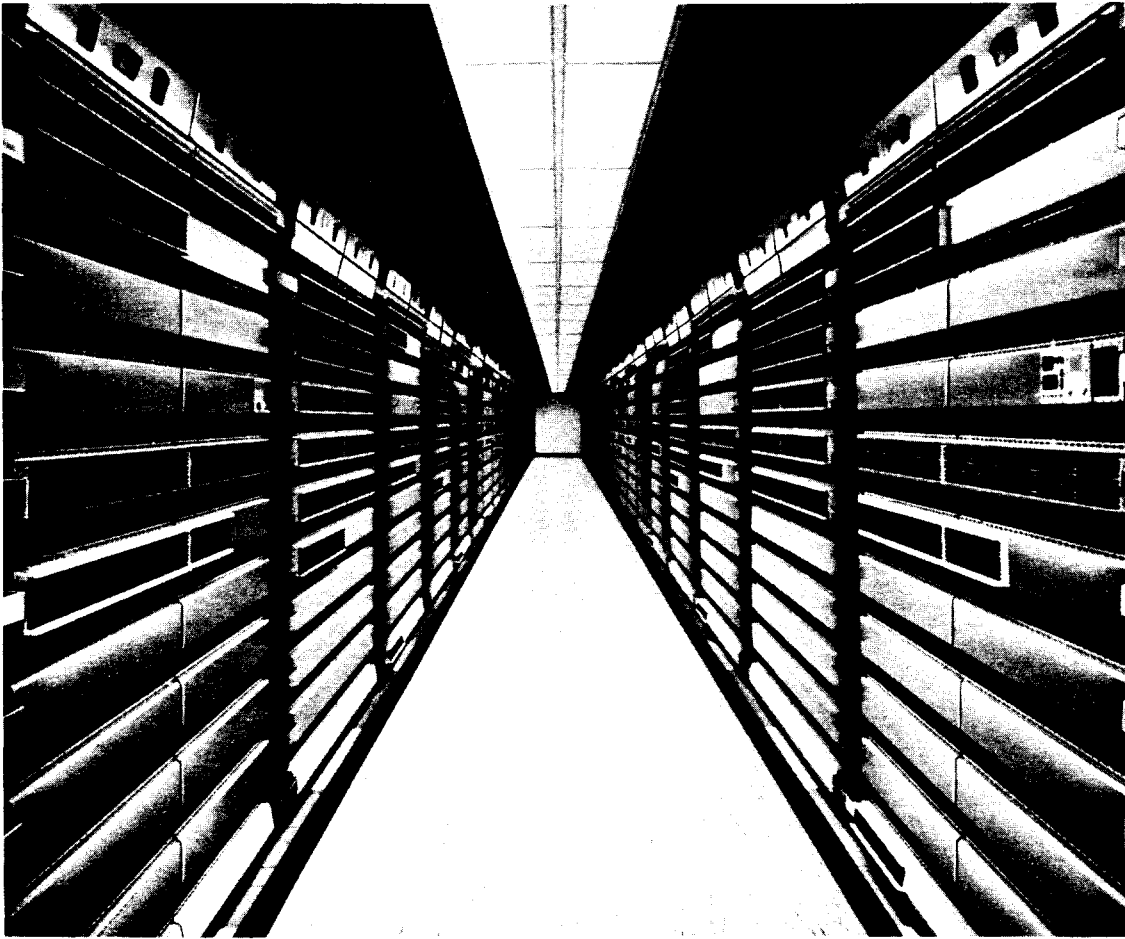
Figure 3-1. COSMIC Distributing Frame System
