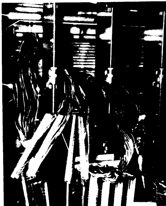
Figure 8-45. Preparing to Press 710 Connectors Together
