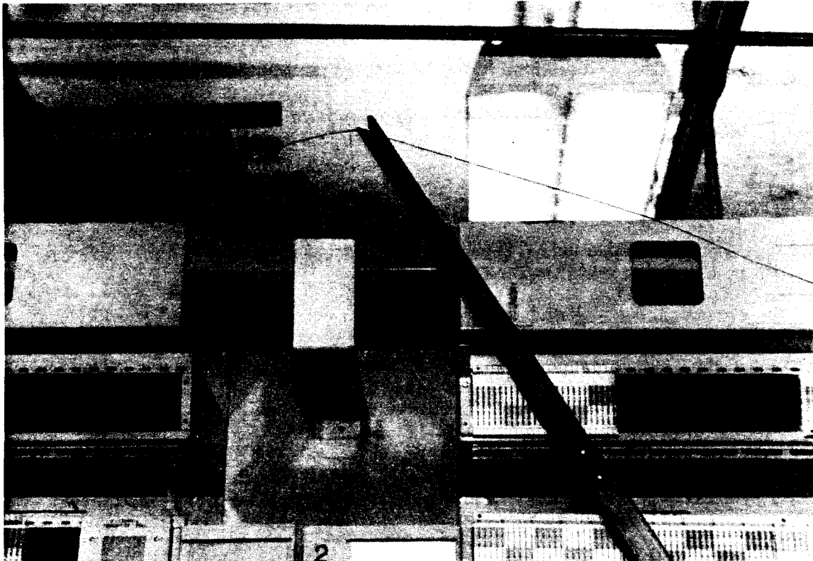
Figure 4-42. Placing Jumper Wire in Trough Using Jumper Running Tool
