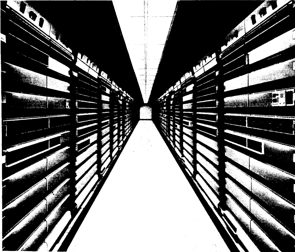
Figure 1-2. COSMIC Distributing Frame System
