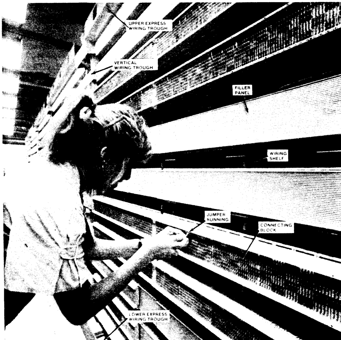
Figure 3-5. COSMIC IIA DF (Front View)
