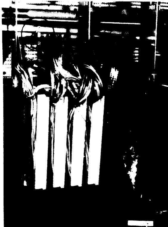
Figure 8-50. Securing Cable Stubs and Connector Ground Leads
