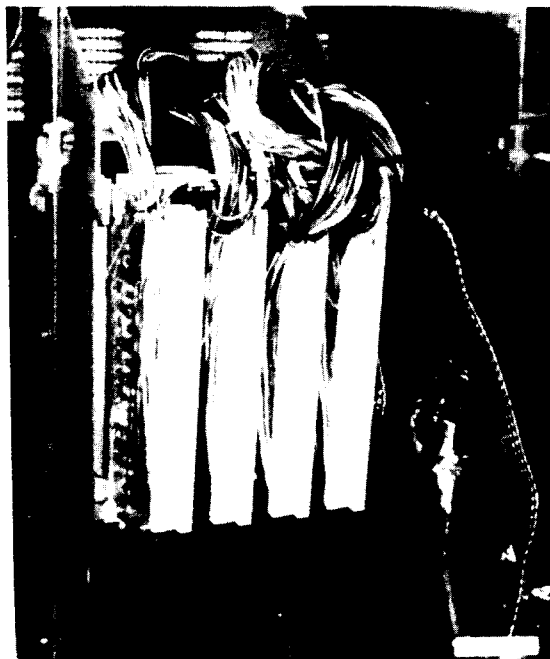
Figure 8-48. Four 710 Connectors Pressed into Position
