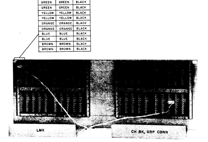
Fig. 2—Type II Group Distribution Frame Cross Connection Panel
