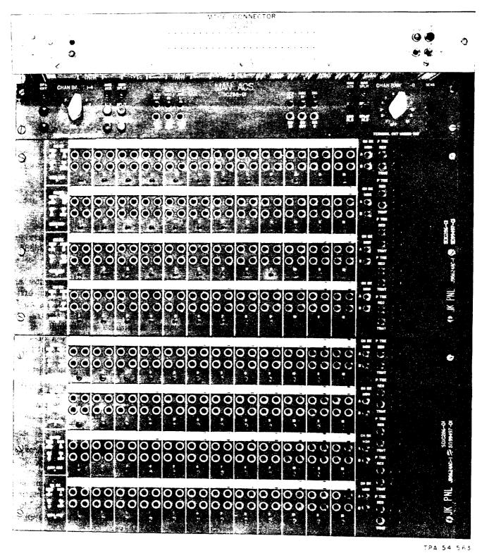
Fig. 3—J98622AA Maintenance Connector, J98622AD Manual Access Panel, and J98624AC VF Jack Panel
