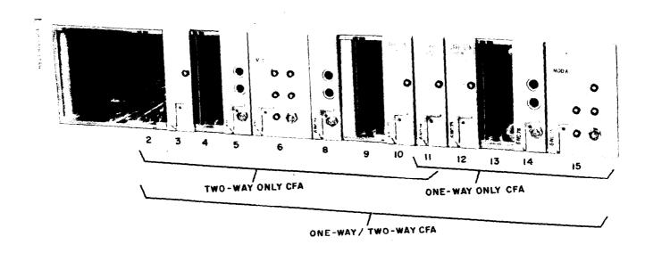
Fig. 5—A6 CFA Carrier Supply Arrangement—J68929( ) Bays and J98626( ) Frames
