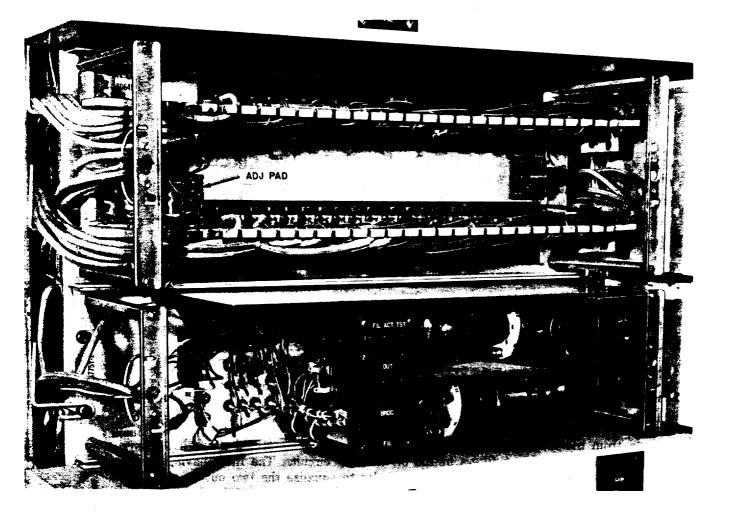
Fig. 1—Group Carrier Distribution Bus and Associated Distribution Amplifier
