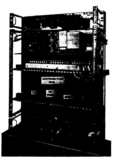
Fig. 1—88-kHz Carrier Amplifiers and Associated Distribution Bus
