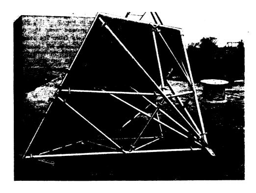
Fig. 3 — KS-16320 Passive Reflector Arranged for Inspection of Surface
