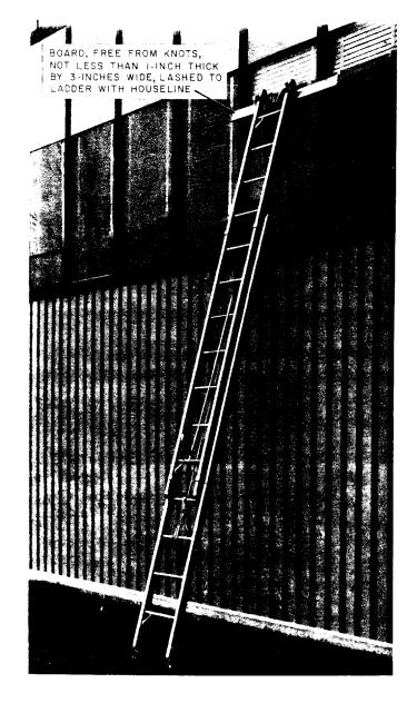
Fig. 17—Ladder Placed in Front of Window
