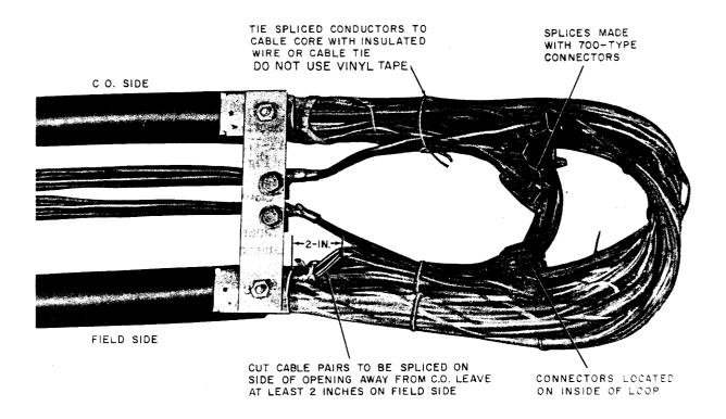
Fig. 6—₱Wire Work Completed—14-Type Closure♥
