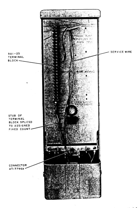
Fig. 12—PService Wire Terminated in PC12/55 Cable Closure—Fixed Count Mode
