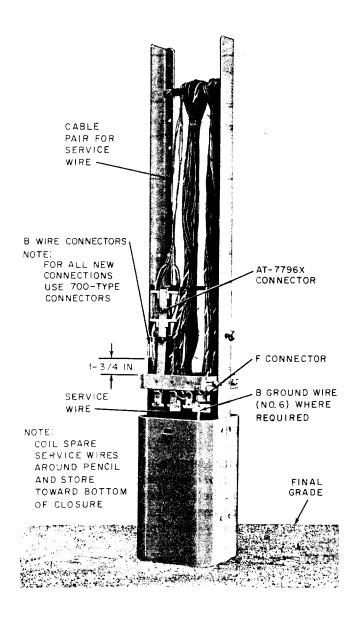
Fig. 20—♦Service Wire Installed—LD Type Cable Closure♦
