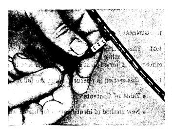
Fig. 2—▶Placing Tie and Marker¶
