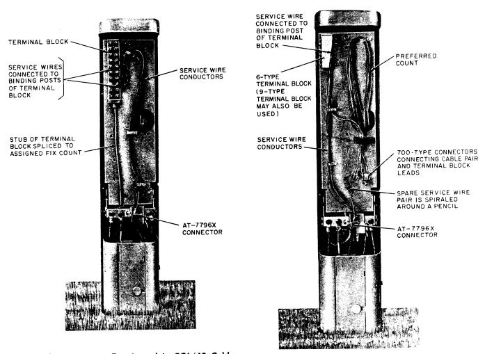
Fig. 10—♦Service Wires Terminated in PC6/48 Cable Closure—Fixed Count Mode♦
