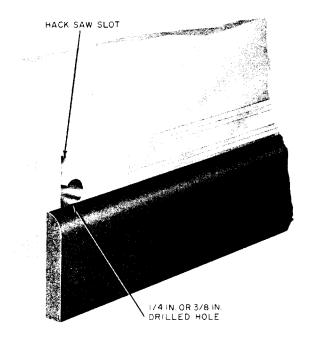
Fig. 15—Hole Through Wall for B Station Wire
