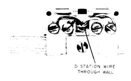
Fig. 6—Terminating Wire on No. 717 Terminal
