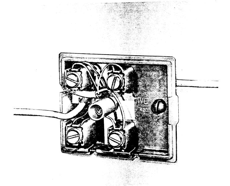
Fig. 2-\$42D Connecting Block Mounted on Wall
