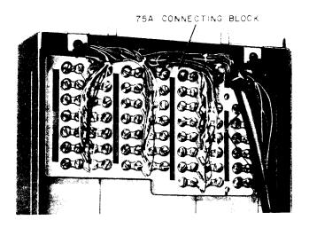
Fig. 6—75A Connecting Block Installed in Apparatus
