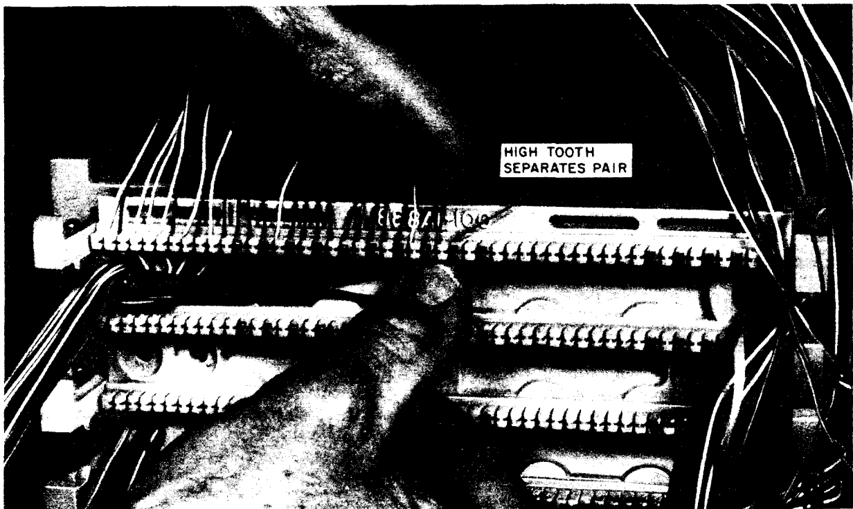
Fig. 17—Placing Conductors in Index Strip
