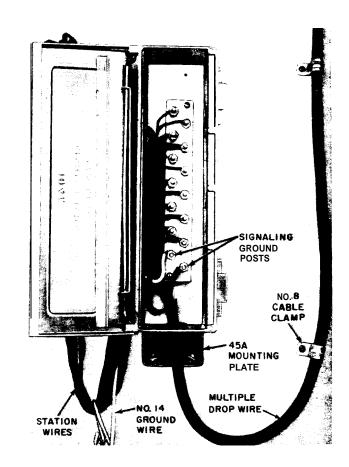
Fig. I-Wiring of 104A Wire Terminal
