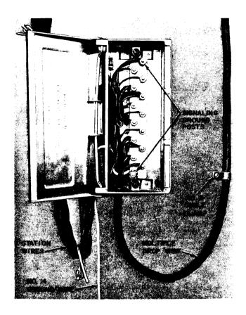
Fig. 2-Wiring of 104B Wire Terminal
