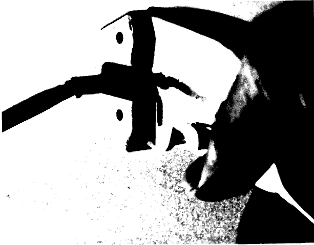
Figure 11 Pressing the U1R Connector for a Dependable Splice
