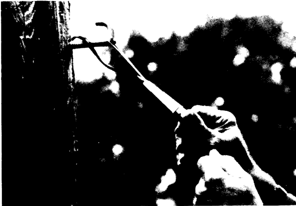
Figure 5 Drop Wire Attachment to Pole
