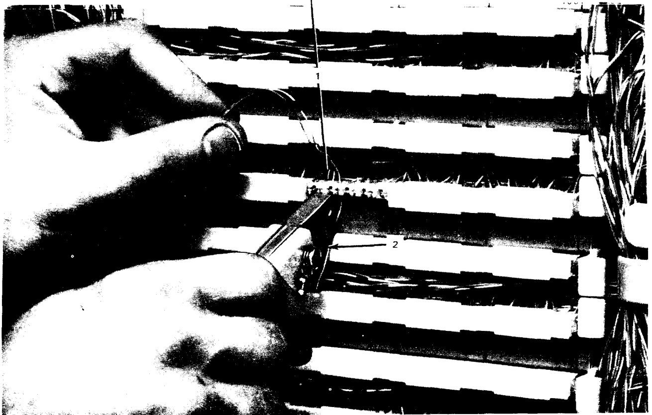
Fig. 5—Terminating Cross-Connecting Wire on Feeder Field
