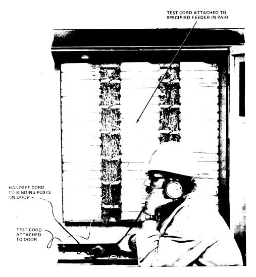
Fig. 3—Verifying Feeder-In Pair—108-Type Connectors
