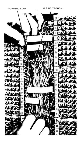
Fig. 11—Forming Finger Loop and Placing Wire in Wiring Trough
