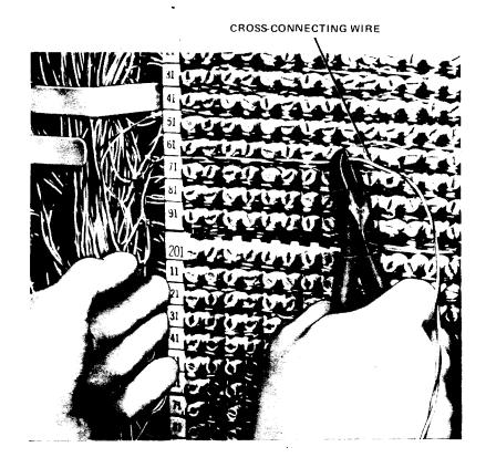
Fig. 12—Cutting Cross-Connecting Wire
