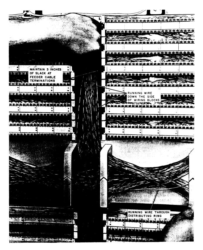
Fig. 4—Positioning Cross-Connecting Wire
