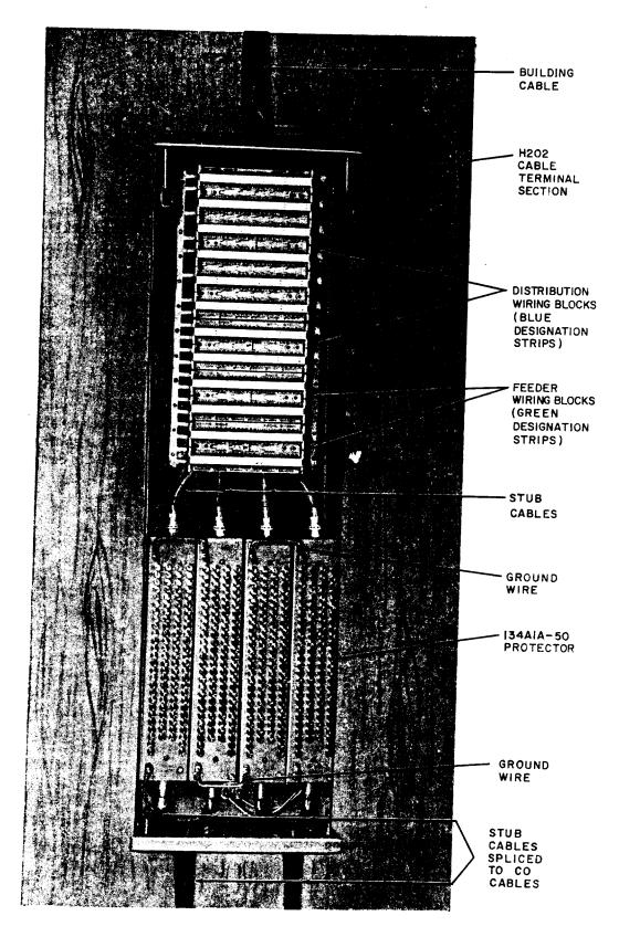
Fig. 7—200-Pair Exposed Entrance Cable—400-Pair Building Cable
