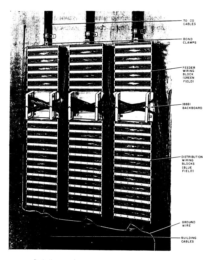
Fig. 1—Main Terminal—900-Pair Entrance Cable—1800-Pair Building Cable
