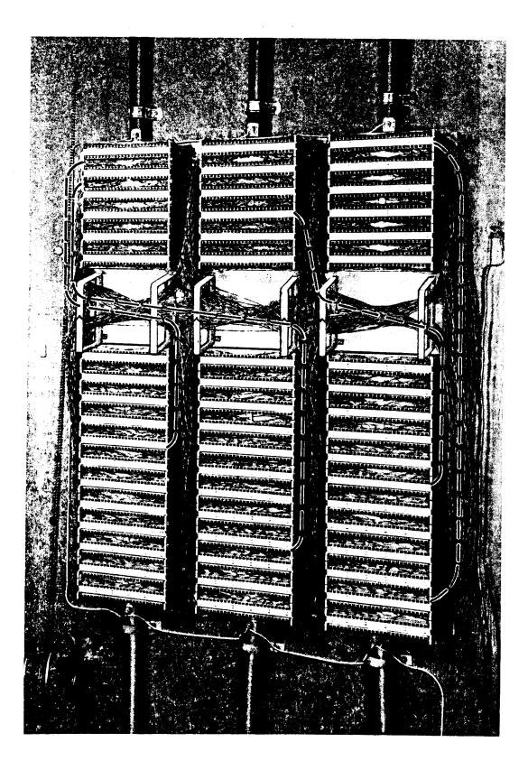
Fig. 5—Various Cross-Connecting Wiring Paths
