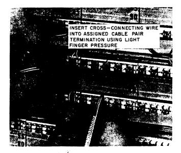
Fig. 2—Inserting F Cross-Connecting Wire Into 88-Type Connecting Block
