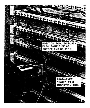
Fig. 3—Seating and Cutting Cross-Connecting Wire Into Connecting Block
