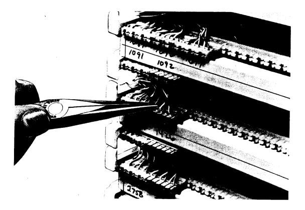
Fig. 9—Removing Cross-Connecting Wire
