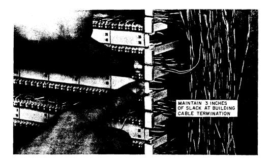
Fig. 6—Positioning F Cross-Connecting Wire to Assigned Building Cable Pair
