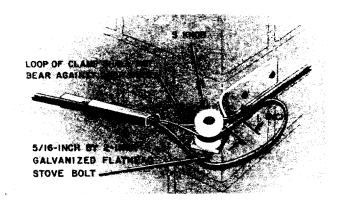
Fig. 13—₱First Attachment—Corner Bracket With S
