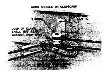
Fig. 11—₱First Attachment—House Bracket (Horizontal Run, Double Wire) With S Knob
