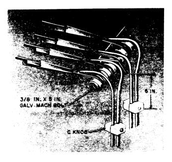
Fig. 8—First Attachment—House Bracket (Vertical Run, Four Wire) With T Knob
