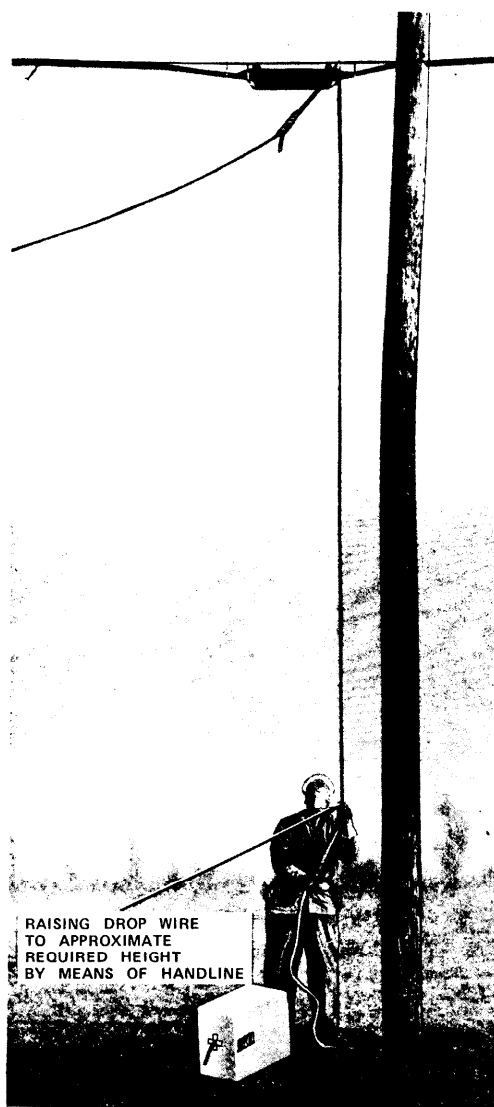
Fig. 8 - Raising Drop Wire - Dispenser Method
