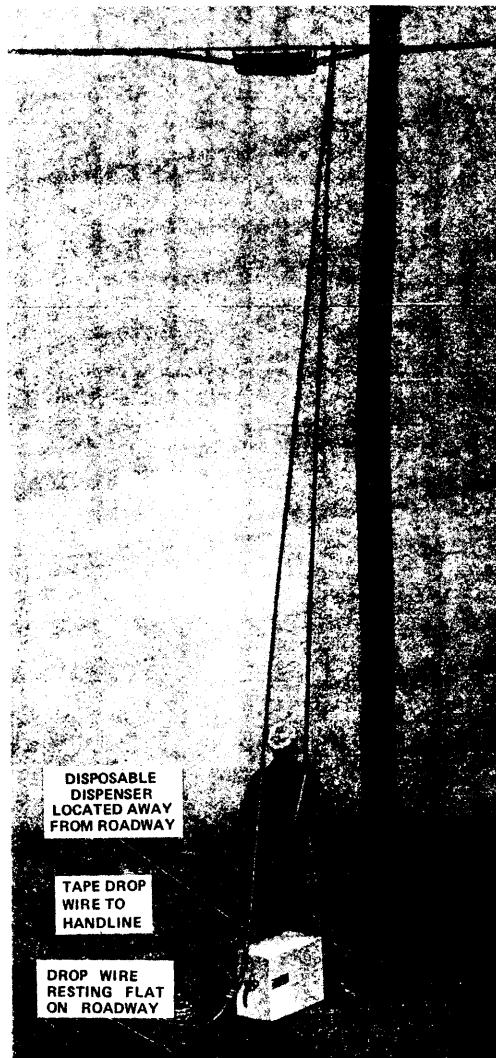
Fig. 5 - Handline Taped to Drop Wire
