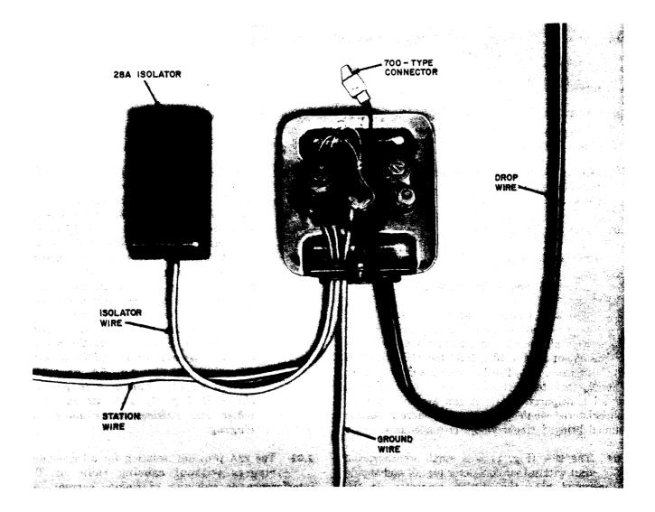
Fig. 1—28A Ringer Isolator, Typical Installation
