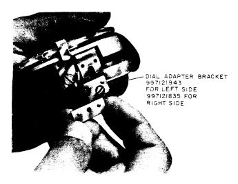
Fig 15—Placing Dial Adapteer Brackets on Rotary
