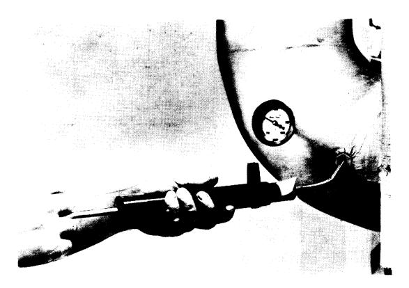
Fig. 11—Taking a Smoke Sample
