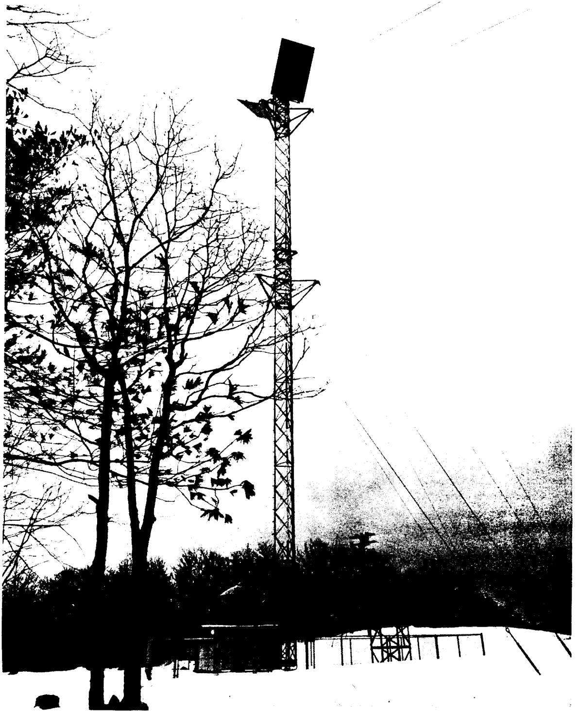
Fig. 3 – A TYPICAL SHORT HAUL MICROWAVE REPEATER STATION — Parabolic type antennas, covered with radomes for protection against snow and debris, are aimed toward reflectors at the top of the tower for transmission of signals to adjacent stations.
